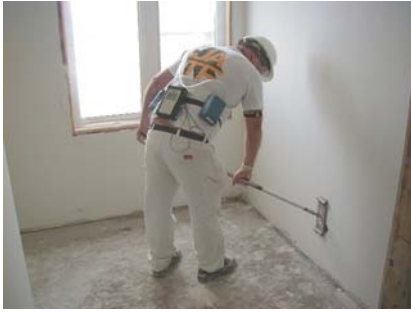
FIGURE 1. Sanding drywall using a pole sander
