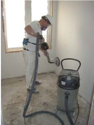
FIGURE 2. Shrouded ventilated rotary sander (SVRS) attached to vacuum
